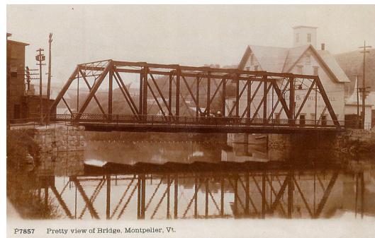
P7857 Pretty view of Bridge, Montpelier, Vt.
